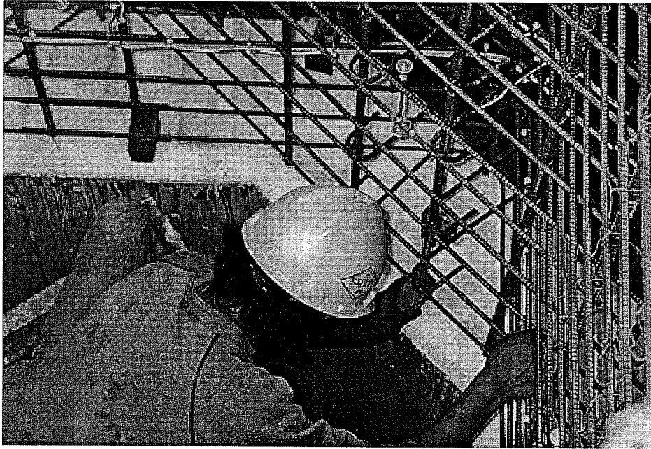
Figure 4.9: Placement of 50 mm thick cinder blocks under reinforcement cage.
