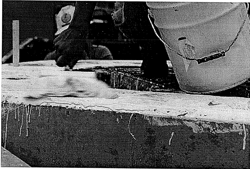
Figure 4.7: Application of bond breaker to bulkhead segment top face.
