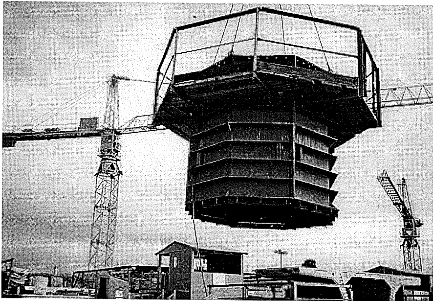
Figure 4.8: Pier segment outer form and scaffolding.
